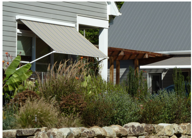
Getting the best performance from your windows may involve both an interior and an exterior attachment. Note the interior shades and exterior awning serving this set of windows.
