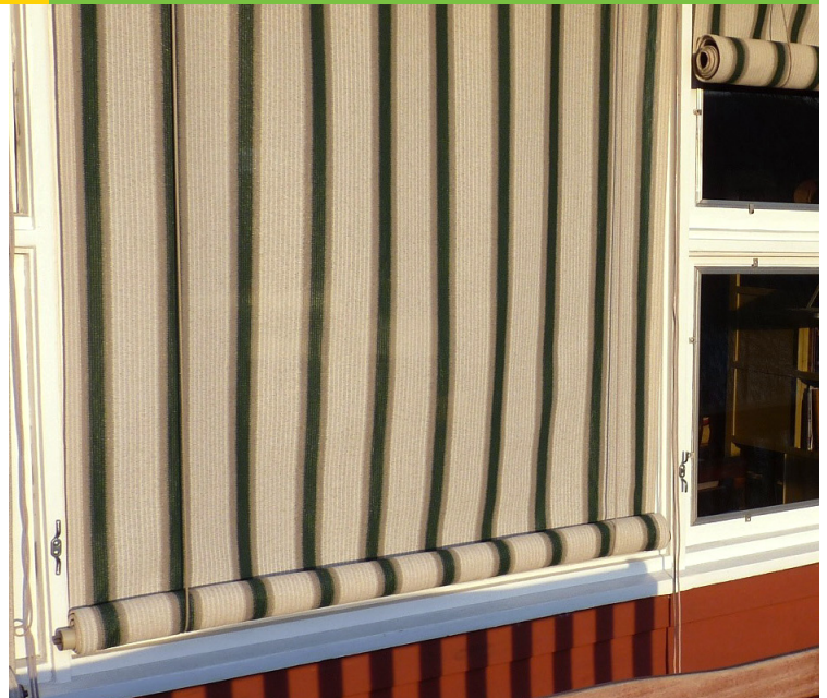
This exterior roller shade is operated manually to control glare and solar heat gain, particularly in the summer (the home is located in New England).
