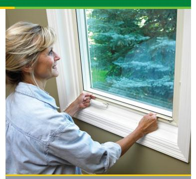
Interior fixed window panels can be plastic or glass. All are fairly simple and inexpensive. Only glass interior fixed panels are available with a low-emissivity coating, which reduces the movement of heat from the warmer side to the cooler side of the glass, saving energy by keeping desirable heat in the home in cold weather and undesirable heat out of the home in warm weather.
