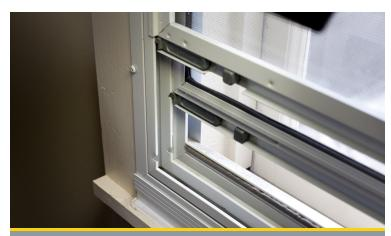
Tracked interior window panels are just like exterior storms, but permanently installed on the inside of the window. With integral screens, they adjust for ventilation. Made of glass, they are durable, clean easily, and are available with low-e coatings.
